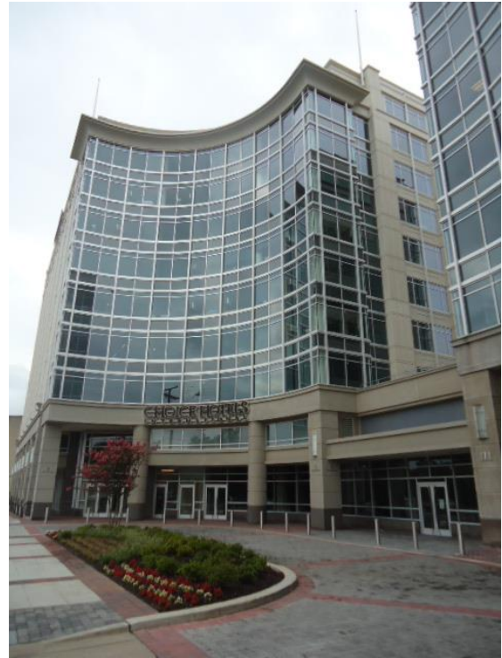
Figure 22: North East Curtain Wall – by JMV
