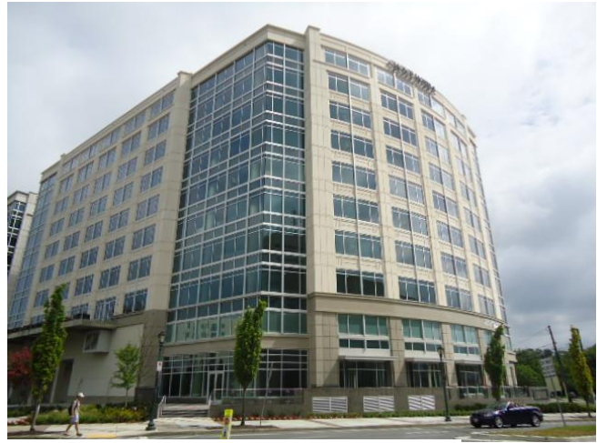
Figure 2: South West Corner – by JMV
