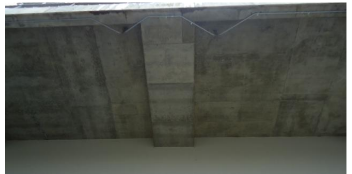
Figure 25: Projection of Post Tension Beam – by JMV
