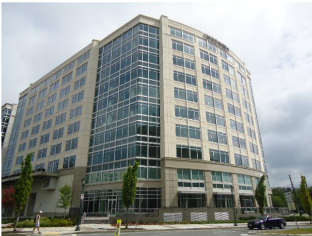
Figure 24: South West Corner – by JMV
